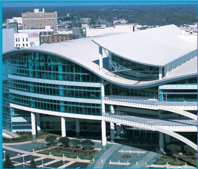
Reflective roofs like this one can help save energy in warm, southern climates, but they are typically not the most efficient option in cooler, northern locations.
