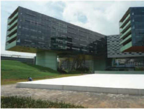
The cable-stay structure permits open facades.
