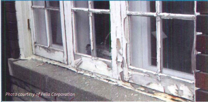
Window deterioration
