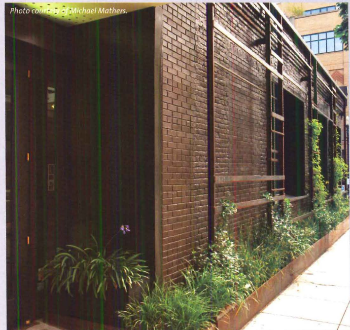
Through water-efficient fixtures and reused rainwater, the AIA reduced its annual potable water demand for toilets and urinals by 97 percent, plus provides for the Center's minimal irrigation needs.
