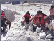
The sandbags are plastered over on the exterior. The bags are dampened beforehand to ensure that the plasterwork cures instead of merely drying (far left). Residents of the township participated in the construction by filling sandbags (left).
