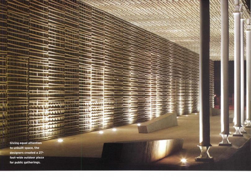
A distinctive feature of the building that required special training to construct was the gabion wall. Nothing more than cages of rocks, gabions are more commonly used in civil engineering projects for erosion and flood control. For the library, experienced road builders from the region were
