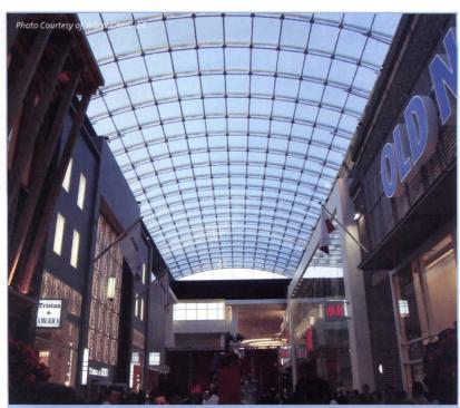
Transparency and performance are both enhanced with an ionoplast interlayer in the glass roof of Yorkdale Mall, Yorkdale, Ontario, Canada.
