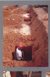
To conform to seismic regulations in this earthquake-prone region, foundations were dug 6.5 feet deep (left). Stones collected from nearby rivers are encased in PVC-coated wire (below left). The west facade is composed of panels of sticklike pieces of pine arranged in a slanted pattern (below right).
