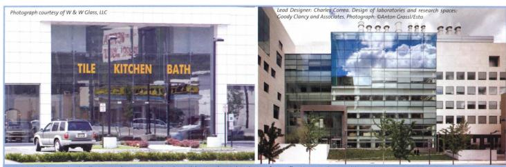
On the left, standard roller wave distortion is clearly visible. On the right, the perfect reflection made possible in glass controlled for roller wave, in the extraordinary bolted structural glazing system on the facade of the Brain and Cognitive Sciences Complex, Massachusetts Institute of Technology, Cambridge, Mass.
