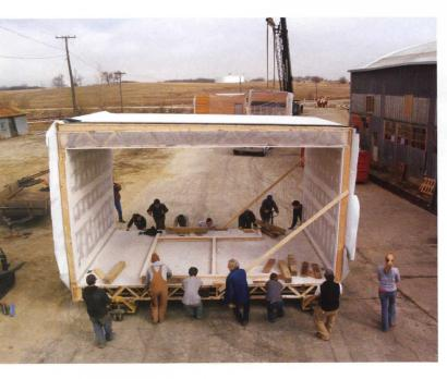
Students prepare to load one of the prefabricated modules of the 5.4.7 Arts Center onto a truck (left); later, it was hoisted into place
