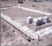
Sand is a cheap, durable, and easily obtainable building material. In this flood-prone area, foundations for the house are lined with sandbags (above). Walls of sandbags offer excellent thermal and sound-absorbing properties (right).
