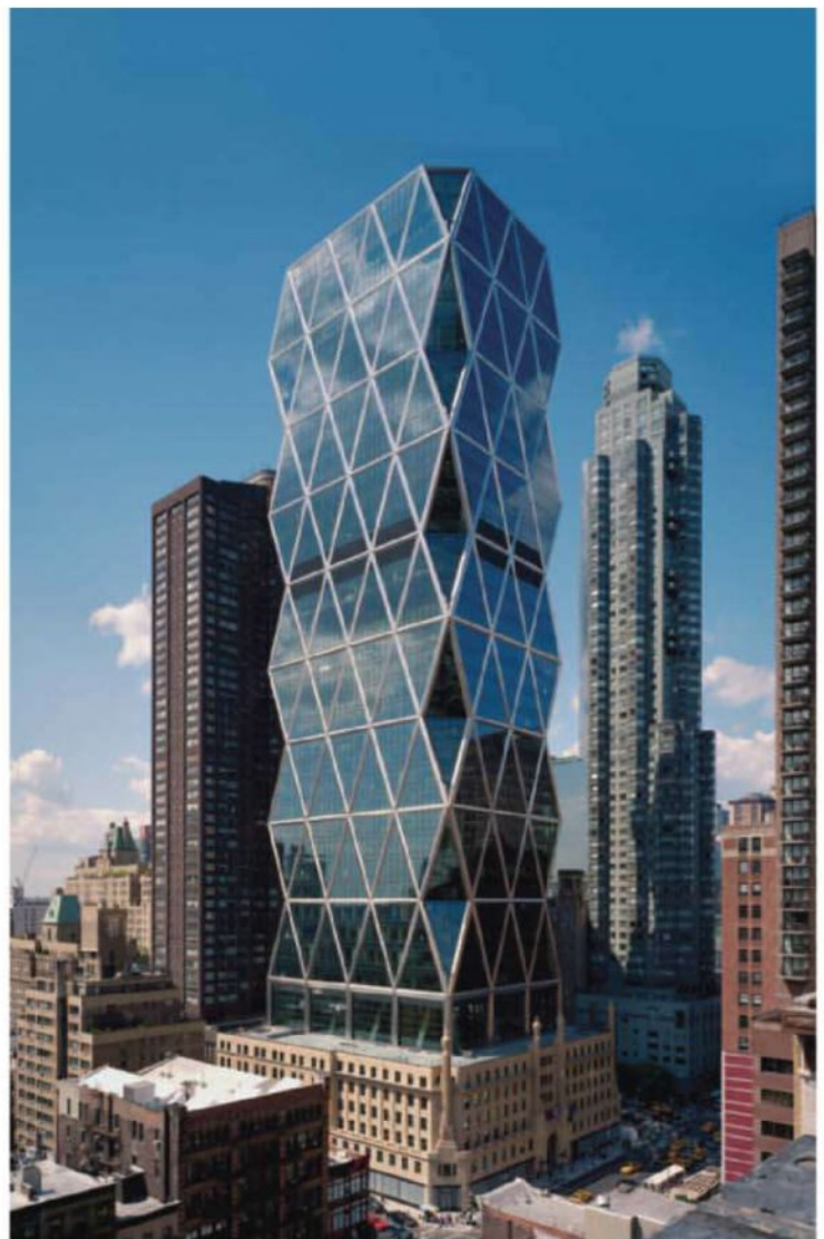
The new Hearst Tower sits on top of a six-story base built in the 1920s.
