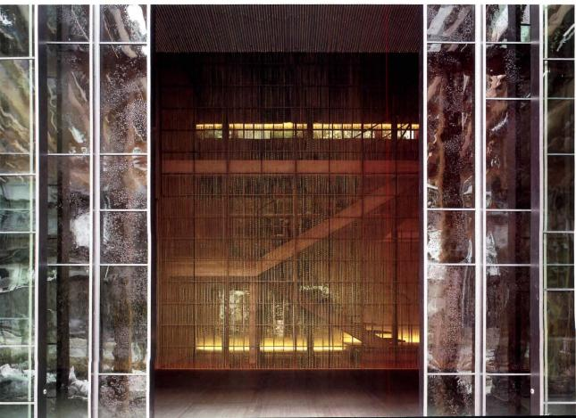
Subtly lit treads suspended from the ceiling on steel rods give a stair connecting the top two floors a sense of floating in space (above). A 700-year-old French handblowing technique called dalle de verre was used to create part of the almost-transparent glass entry wall (left).
