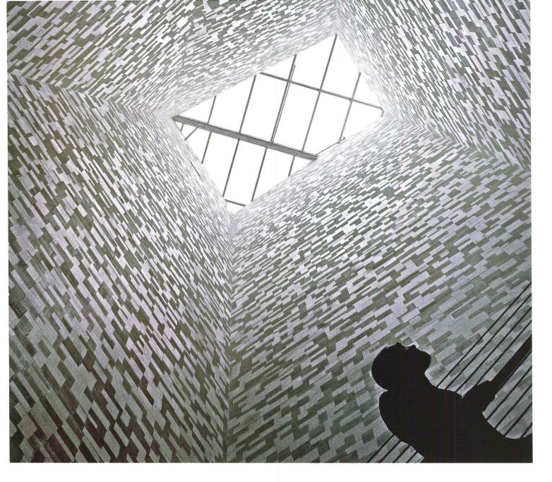
second light well extends from what is called Level 5 to Level 6 before becoming an enclosed shaft puncturing the roof. The third light well is totally enclosed; a fire stair winds through its skylit core, also finished in hand-notched plaster. The effect is mesmerizing.
