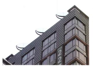
At Battery Park City's Teardrop Park, Carpenter Norris Consulting installed three heliostats (left and below two) to bring daylight into a secluded urban landscape. The mirrors track the sun and reflect elliptical-shaped spots of daylight-at nearly 90 percent of the sun's brightness-onto eighteen places in the park. Alternately, fiberoptic cable (bottom) is used by Parans to bring daylight to otherwise conventional-looking light fixtures deep within a building.
