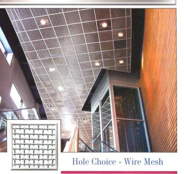
Wire mesh panels used for this ceiling grid are aesthetically pleasing and have functional properties, such as air and light diffusion along with accurate acoustical benefits.
