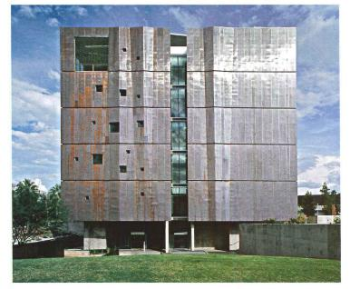
The lab building (above), depressed slightly below grade, features an outdoor sitting area at the glazed base of the gleaming copper cube.
