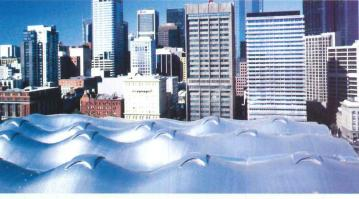
**Grimshaw Architects'** design for the Southern **Cross Station in** Melbourne, Australia, takes advantage of crosswinds to induce the stack effect in a double-skinned domed roof. The architects and engineers relied on 19th-century trainstation designs to inspire the completely naturally ventilated station, since computational fluid dynamic modeling could not be undertaken until design had progressed significantly. The station, open since 2006, has been considered a success.
