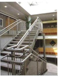
P & P Artec Modesto system, has 1 single round baluster. All fittings are powder coated. Their other systems include the Chicago – (flat bar baluster). Double Baluster – (2 round balusters), and Munich – (3 oval baluster). Artec has build a reputation in 100% seamless handrail tubes. All of their systems are assembled and finished in the field, to provide each project a unique custom installation, without any visible joints.
