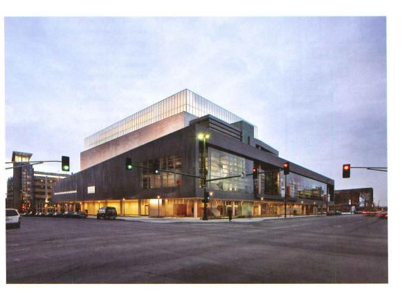
The second-floor lobby "floating wedge" is clad in zinc panels, while the box of the concert hall is limestone with a glass clerestory (left). The ground floor's glass curtain wall, supported by thin fins, creates a "see-through" effect for the Holland's public spaces.
