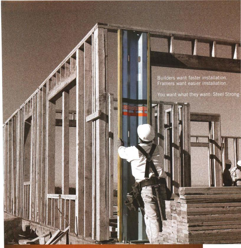
Specify Steel Strong-Wall<sup>®</sup> by Simpson Strong-Tie and you'll also get what you want without sacrificing your design. By combining steel and wood, Steel Strong-Wall makes it easy to achieve high loads in narrow spaces. Steel Strong-Wall is available in five widths from 12 inches to 24 inches and heights ranging from 7 feet to 13 feet. For more information on how Steel Strong-Wall can work for you, visit us at www.strongtie.com or call 1.800.999.5099.
