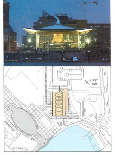
immense conical funnel that tapers up through the glazed pavilion to pierce a hovering roof plane. Ripping and swelling like a shaken carpet, the contoured underside of the roof is lined with thin strips of untreated red cedar. Slender steel columns support the undulating roof as it extends beyond the Miesian glass box to form a dignified and welcoming colonnade.
