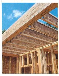
iLevel<sup>™</sup> Trus Joist® Parallam® parallel strand lumber (PSL) is known for uniform quality, strength and good looks. iLevel's revolutionary technology delivers beams, headers and columns that are stronger, straighter and longer than conventional lumber. Parallam PSL beams and headers are available in large sections, eliminating field assembly and are compatible with common hardware—making installation quick and easy.
