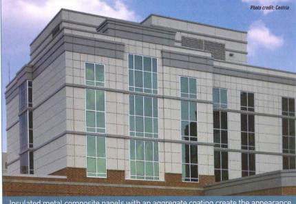
Insulated metal composite panels with an aggregate coating create the appearance of pre-cast on the exterior of the Parkwest Medical Center in Knoxville, TN.
