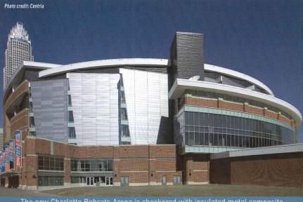
The new Charlotte Bobcats Arena is checkered with insulated metal composite wall panels in custom shades of gray for an original appearance.
