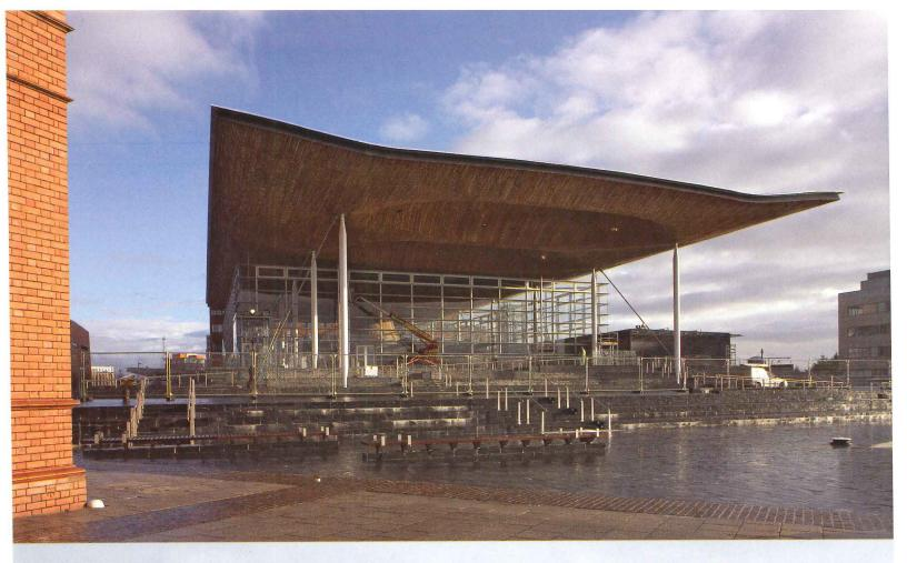
The building's steel roof incorporates six elliptical domes, with one topped by a lantern and a 20-foot-tall, rotating wind cowl (above and below). An iconic funnel above the debating chamber is visible at night (opposite).
