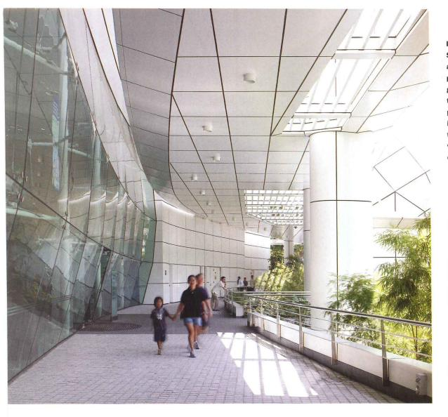
while the latter controls temperature by chilling interior spaces, albeit at the expense of energy efficiency. In his design for the National Library, Yeang explores a third way—harnessing cooling breezes, sun-shading devices, daylighting strategies, and planted terraces and skycourts to create a building that is both transparent and ecofriendly.
