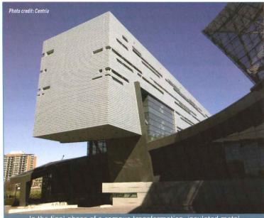
In the final phase of a campus transformation, insulated metal composite panels on the exterior of the housing building help create the new focal point of the University of Cincinnati campus.
