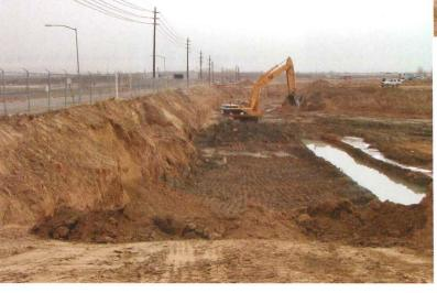
Parsons' contractors scraped nearly 5 million tons of soil, both contaminated and clean, from the surface of the abandoned Stapleton International Airport. In some areas, contractors dug down as far as 25 feet. Once the 3-to-5foot-deep "smear zone"
