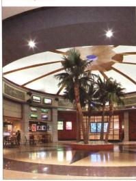
Backlit suspended frame and fabric ceiling panels. Just one example of the numerous custom solutions provided by Eventscape. Designers have the freedom to create virtually any form, clad with any material. Custom ceiling solutions engineered and fabricated to meet your specifications. View their complete portfolio on their web site. Create without boundaries.
