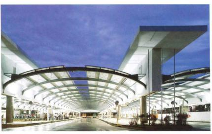
The roof of Nucleo de Arquitetura's Lapa Bus Terminal expels exhaust while filtering sun.
