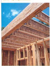
iLevel™ Trus Joist® Parallam® parallel strand lumber (PSL) is known for uniform quality, strength and good looks. iLevel's revolutionary technology delivers beams, headers and columns that are stronger, straighter and longer than conventional lumber. Parallam PSL beams and headers are available in large sections, eliminating field assembly and are compatible with common hardware—making installation quick and easy.
