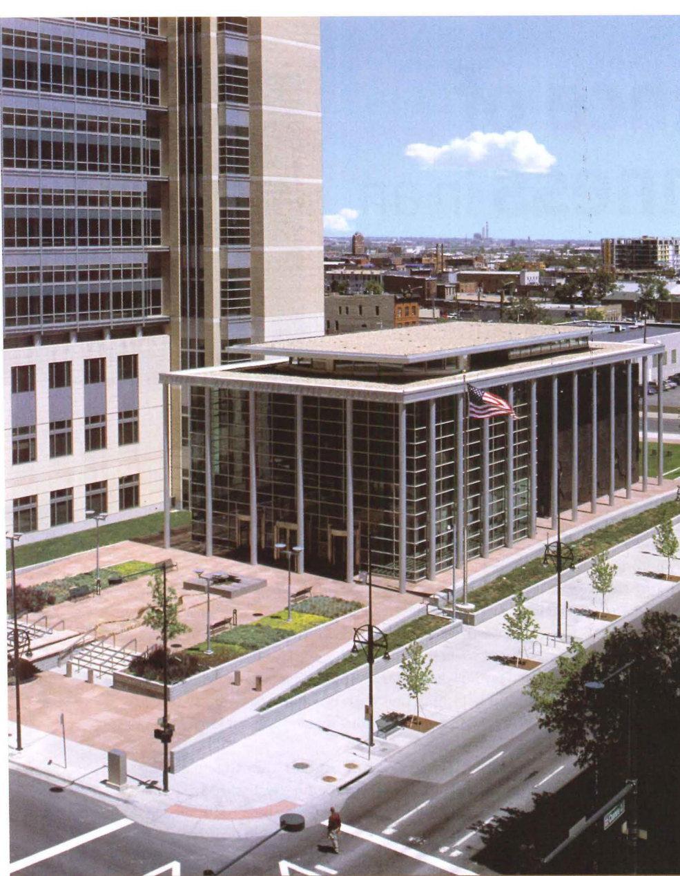
At the Arraj Courthouse, the plaza and lobby pavilion are publicly welcoming, yet discourage vehicle bombs and limit a terror attack's damaging effects.
