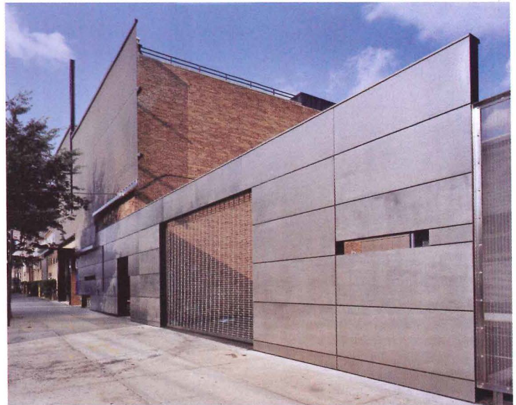
The brick facade and parking court (left) was covered in a grid of bead-blasted stainless-steel panels with Z-clip reveals (above). A stainless-steel-mesh screen is hung from the second-story roof (opposite).
