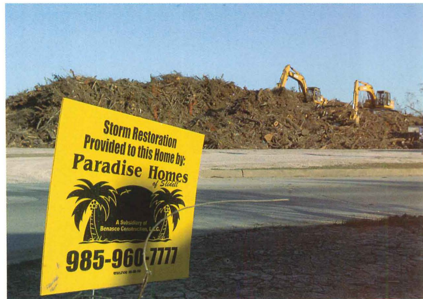
Orange waterlines are sometimes the only clue to the devastation inside homes and buildings. Canal Boulevard, near City Park, has been turned into a giant trash dump.
