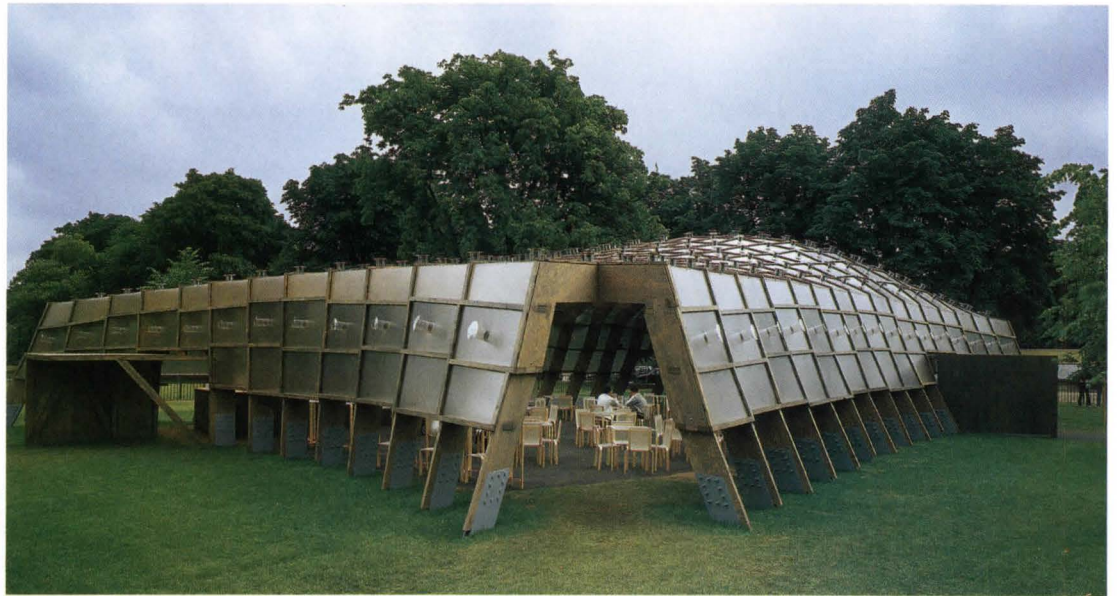
Interlocking timbers of 427 different lengths (above) create a column-free interior 56 feet wide (below).
