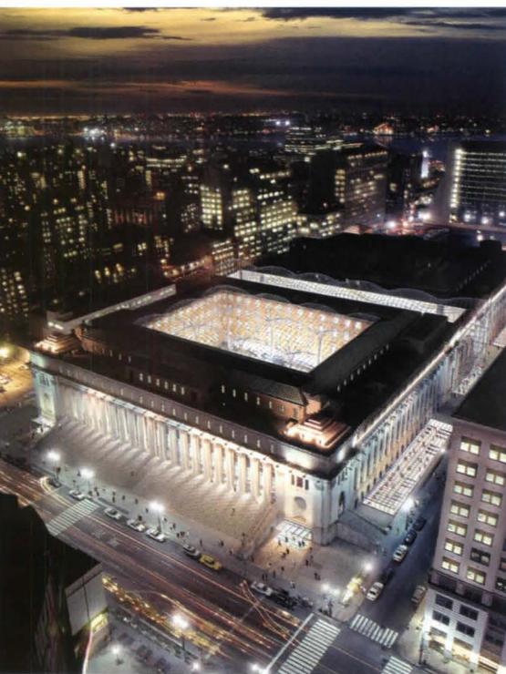
The Beaux Arts-style Farley Post Office will become a train station. "Light moats" along sidewalks will bring natural illumination underground.
