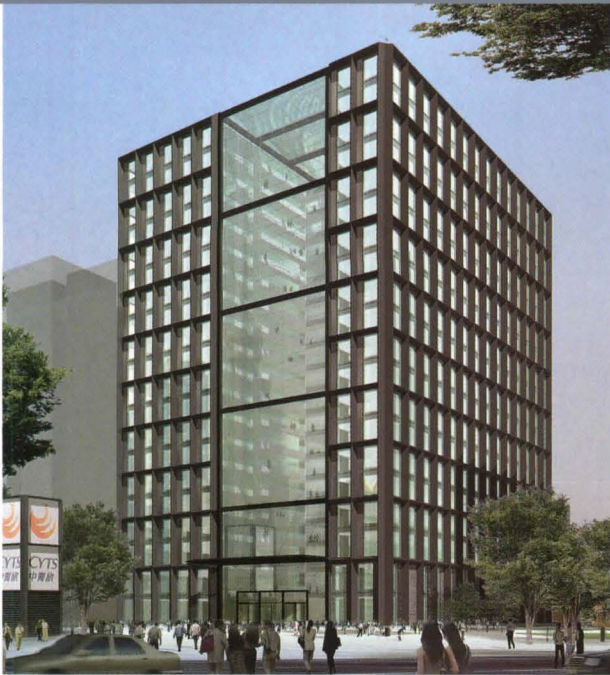
CYTS Plaza in Beijing Designed by von Gerkan, Marg and Partners and Arup Hong Kong, the 22-story tower (scheduled to be completed in December) will have a vertical band of louvers in the exterior facade covered by a side-hinged panel on the interior facade, which individual users can open and close for fresh air.
