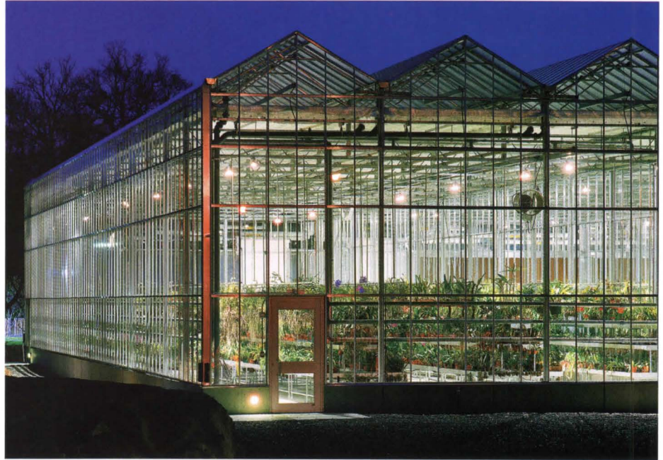
The Nolen Greenhouses at the New York Botanical Garden have state-of-the-art HVAC systems.
