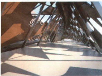
The bridge will be composed of overlapping space frames.
