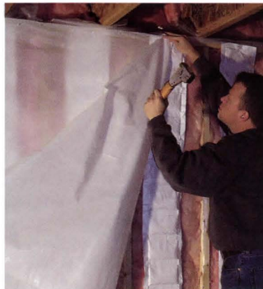
The strips are covered with vapor retarder.
