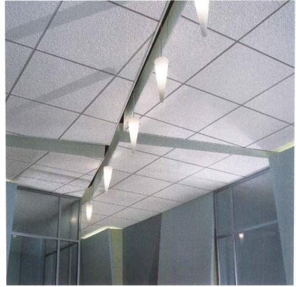
Many acoustical ceiling panels are made from mineral wool, gypsum and smaller amounts of paper and starch, as well as other miscellaneous materials. The mineral wool is made from slag, a by-product of steel manufacturing that consists of calcium silicate and other impurities.
