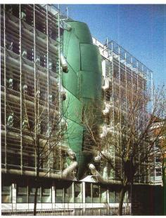
The HVAC system for Arup's new campus on Fitzroy Street in London is clearly visible through a double-glazed curtain wall (left), with ducts and louvers mounted in the plenum space (far left). The ducts meet in the bright green "hub" (left and below), where air enters and exits.
