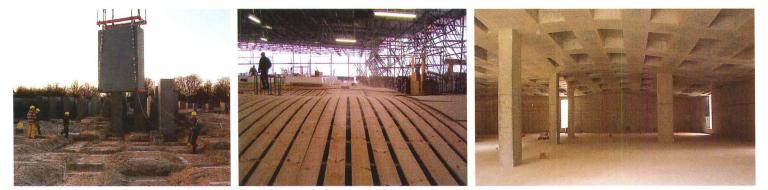
Each stele was lowered into place with a crane (left). Formwork for the coffered ceiling (middle) followed the site's lines, and the concrete was left uncoated (right).
