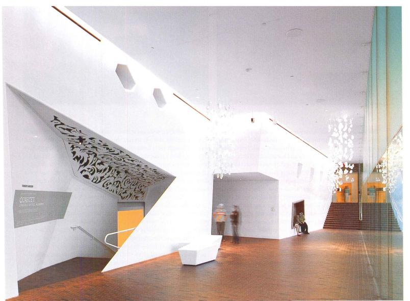
The new galleries (right), like the original ones, are all white with terrazzo floors and parallel ceiling beams. Whereas Barnes chose concrete beams, Herzog & de Meuron used steel members, alternating with conduits. The airflow system for the new galleries also involves the intake vents, hidden behind tracery in the vestibules.
