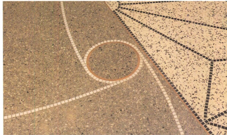
The NTMA establishes national standards for all terrazzo floor and wall systems.
