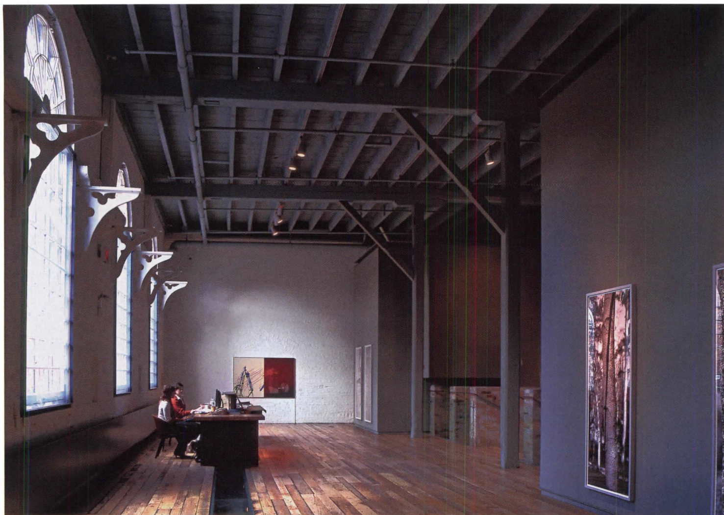
The gallery's reception desk sits in front of three original Palladian windows (above). Old-growth wood flooring was removed, refurbished, and relaid. Restored skylights illuminate the upper-level galleries (right).
