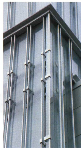
Steel wind clips and staggered shelves hold the glass channels in place (above), and a layer of shiny aluminum siding sits behind the glass.
