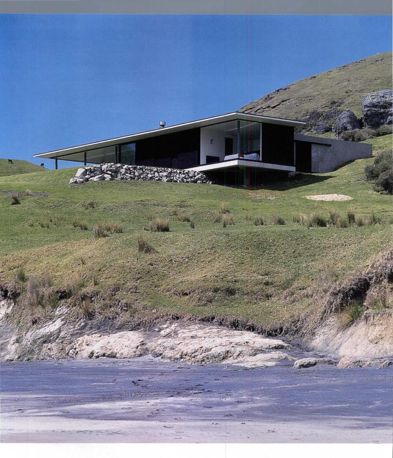
The house is sited along a remote and craggy cove, just where a steep slope levels off into flat, grassy terrain extending out to the surf (above and opposite). The master bedroom, at one corner of the building, cantilevers off the ground. The structure also sits on a low wall of stones, collected from the site (above).
