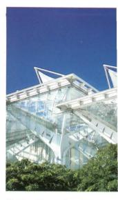
The Hawaii Convention Center, Architect: Wimberly Allison Tong & Goo. Design and Planning: LMN Architects. Features the largest suspended glass wall in the U.S. fabricated by Oldcastle Glass<sup>®</sup> in Stackwall."
