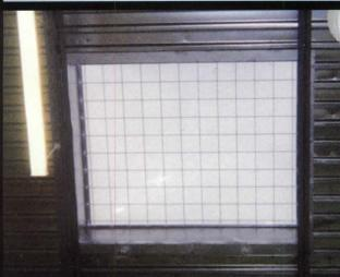
OSHA approved! Interior Safety Screen mounting, instead of exterior mounting, eliminates additional jobsite labor because the screen is built into the RPI structural curb. Saves cost, provides clean exterior look, and offers maximum security against entry. Curb can be manufactured to any bar joist spacing, which eliminates reinforcing. RPI can also supply the skylights, or, just the screens to be mounted inside existing curbs.
