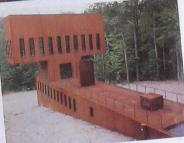
The IIA-inch-thick steel exterior belt was prejabricated in siz parts and then transported to the site, where it was assembled on top of concrete foundations (photo below left). The steel's wickel and dramaion finish has axidized to a vibrani rust color.
