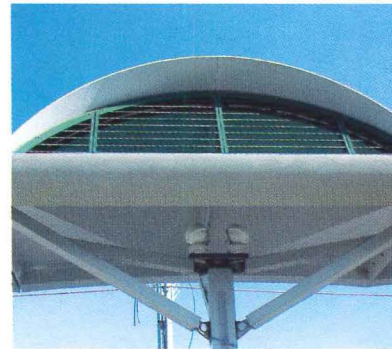
Ductal composite, Lafarge N.A. Concrete & Masonry, page 292.
