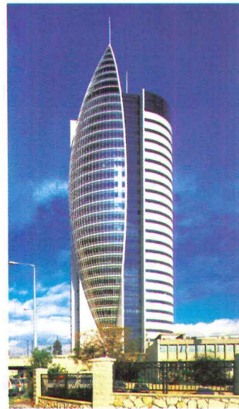
Government Building, Haifa, Israel. Architects: Amar-Kuriel. Features our high performance Energy Absorbing Cable Catch System (EACCS) with blast-resistant laminated glass.
