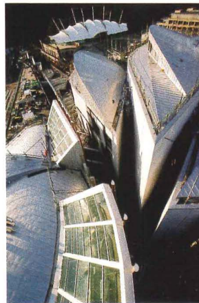
Miralles's structure from above.
