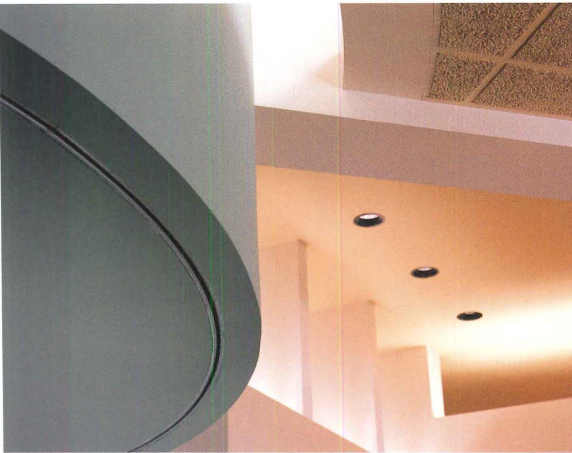
Gypsum is the primary raw material used to make gypsum panels, which score extremely high on nearly all sustainable design criteria. Most of the remaining materials in gypsum board consist of paper and corn or wheat starch binders.
