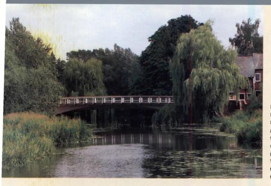
**Ballingdon Bridge** by Brookes Stacey Randall has a complex geometry that required the architects to cut sections through the piers every 2 inches. The final form was tested by rapid prototyping at the University
