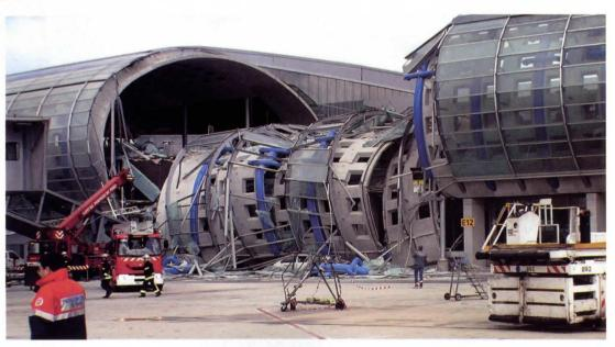
The collapsed area of the concourse is near an "isthmus" link to the main terminal building (seen in center background).
