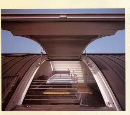
The operable skylight of this London apartment by Brookes Stacey Randall (left) is made of aluminum to reduce the load on the hydraulic openers. The section was manufactured off-site and lifted into place by a crane (far left).
