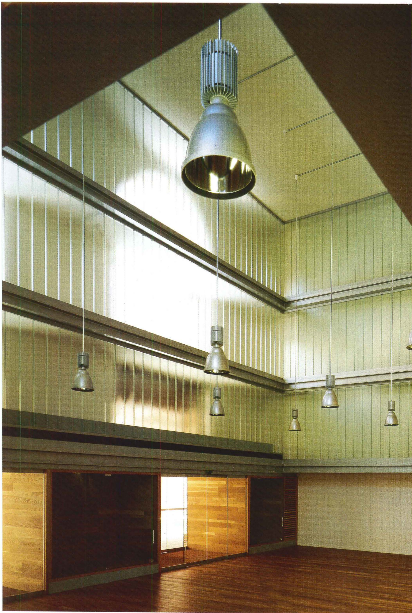
The library's lobby (left) is a three-story volume ringed with the same U-glass used on the exterior of the buildings.
