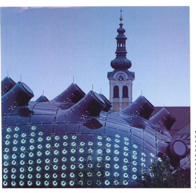
The multisnouted blob, in which a doublecurved, fluorescent-lit acrylic-glass structure is supported by a triangulated steel shell, strangely fits into the the picturesque gableand tile-roofed city. The nozzles are directed north to bring natural light to the exhibition space within.
