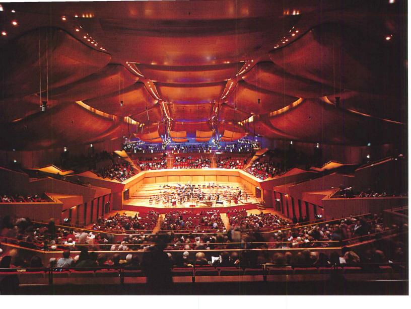
Piano placed the orchestra platform midway between the center and rear of the symphony hall (above), allowing for a tier of seats behind the performers. In addition to clustered ceiling hulls (detail, near right), angular side walls and balconies (far right) play both visual and acoustic roles. This relatively shallow hall was contoured to compress a clear, bright sound and distribute it evenly, all the way to the most distant seats.
