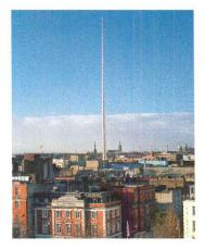
foundries and fabrication shops went into the design, said Robin Cross, the project architect. The spire is built cantilevering into the ground with dampeners to absorb the shock from the structure's movement, which can range up to 3 feet at the apex. The reflective steel is also designed to shift its visual character with subtle changes in daylight and cloud patterns.
