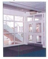
In response to the changes in the IBC 2003 and NFPA 5000 building codes, General Glass International has introduced Pyroshield<sup>™</sup> Plus, a laminated polished wire glass manufactured by Pilkington Glass UK. It is the most cost-effective 45 minutes fire-rated glass including hose stream and has been approved for safety glazing in CPSC Category I applications. For further information call 800.431.2042 Ext. 227.
