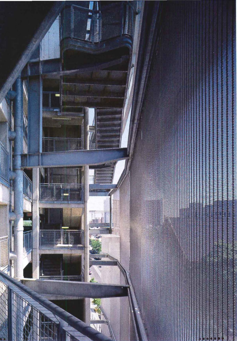
Stairs and ramps pulled away from the bulk of the 765-car garage work with metal mesh and glass
