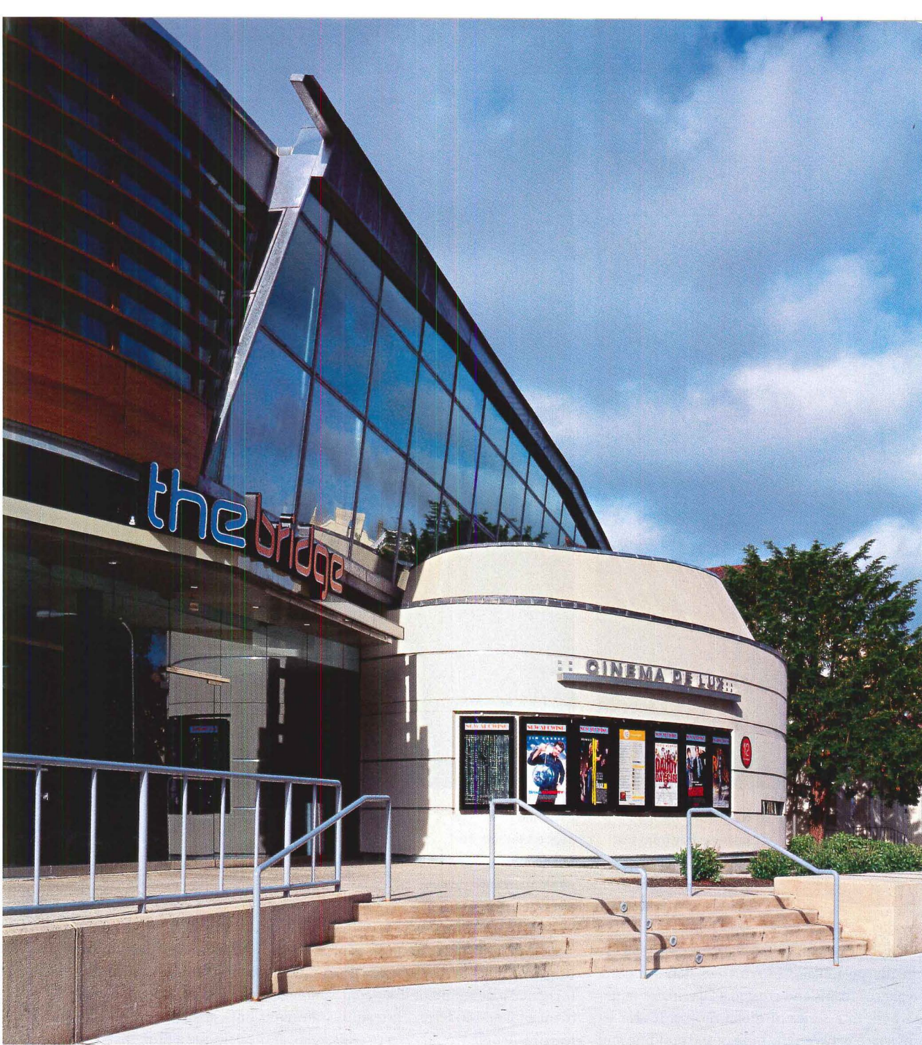
The architects wanted to wrap the curving element protruding from the cinema's main entrance in mahogany and glass, but the new tenant used stucco instead (left and opposite). Daylight and outdoor connections are important elements in both the cinema lobby (bottom left) and the café (bottom right).
