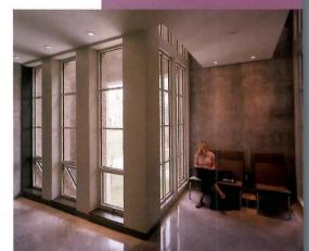
Mexican brick on th **Trustee Hall's north** facade is punctuate by clusters of tall, n row windows (left). 1 fenestration relieves the volume's potenti blockiness without destroying its sense weight and mass. Th hall's central stairca appears through a large, multistory wir dow (center at left). The interiors (below are extremely spare with polished concre floors and exposed concrete columns. Small seating niche along the corridors provide places to re-
