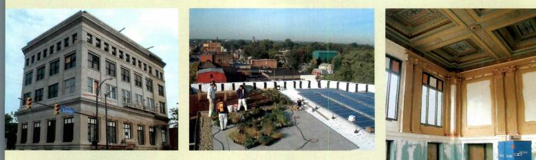
The Cleveland Green Building Coalition bought a 1918 bank (above left) and renovated it using many sustainable features, including a green roof (above center), solar panels, a geothermal system, and waterless urinals. A radiant heat system was installed in the 26-foot-high lobby (right).
