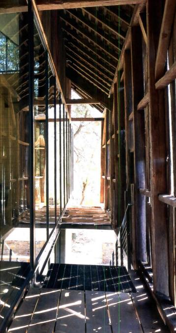
Stock planks, ancho on threaded rods, fo the central service core (top row). Part of the barn's original interior has been fu ther enclosed, in gla while other areas has become more expose as in the entry zone where a new steelgrate stair ascends beneath exposed fla joists, arriving in a semi-outdoor porch (left). The glazing accentuates the pla of light penetrating slots in the cladding (opposite).
