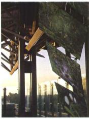
Merrick Architecture At 240 meters, the Lougheed Station (this page) is the Millennium Line's longest. Partner Roger Bayley, a structural engineer, evoked the indigenous rain-forest canopy, held aloft by the longest spans of any station. Three-dimensional trusses stretch as much as 80 meters between clustered columns that like Gothic spires—unite to pierce the gently curving, metal-shingled roof. Art by Danny Singer (above) evokes a sea-to-mountains journey.
