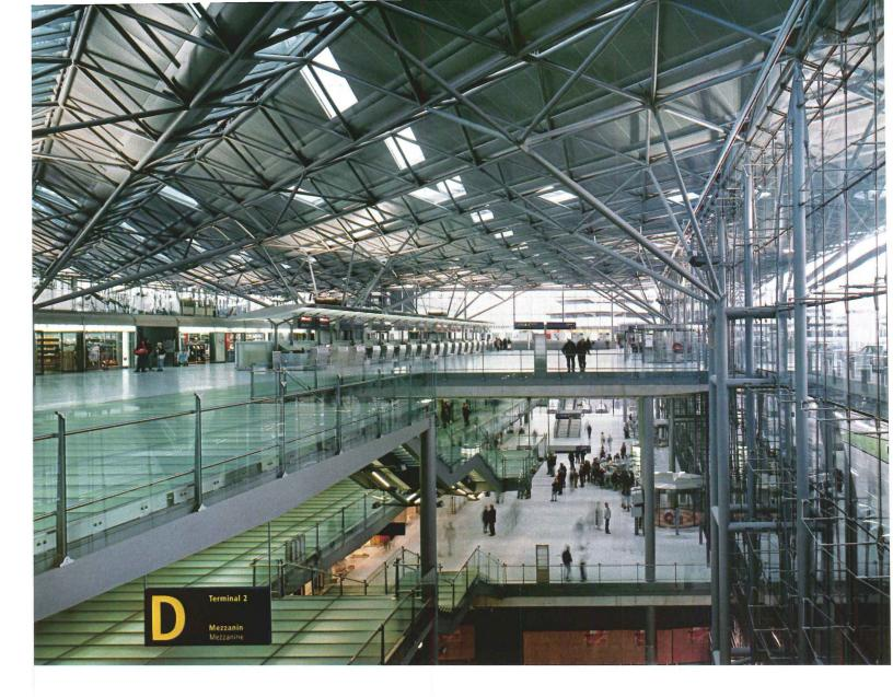
of plate. Terminal Two can be iderstood as a simple glass shed, it also as a laterally expandable ir, 985 feet long and 246 feet ep, built with prefabricated, modar parts. The physical connection itween the two terminals, with ich disparate structural systems, smartly limited to a two-level ass-and-steel bridge.
