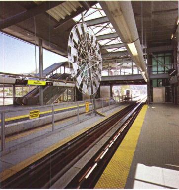
Columns branch into cantilevers to support twin, arching canopies (above). A second, higher canopy echoes the lower with inverted arches that cover the upper entry (top). easy reach of vandals resulted in a number of hybrid structural systems that became what Hart describes as "dialogs of steel and wood."
