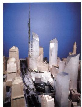
The most dramatic component of his plan includes a memorial space set some 70 feet below grade on a bedrock foundation with the exposed slurry wall on the west. An elevated walkway encircling the site constitutes a memorial promenade.
