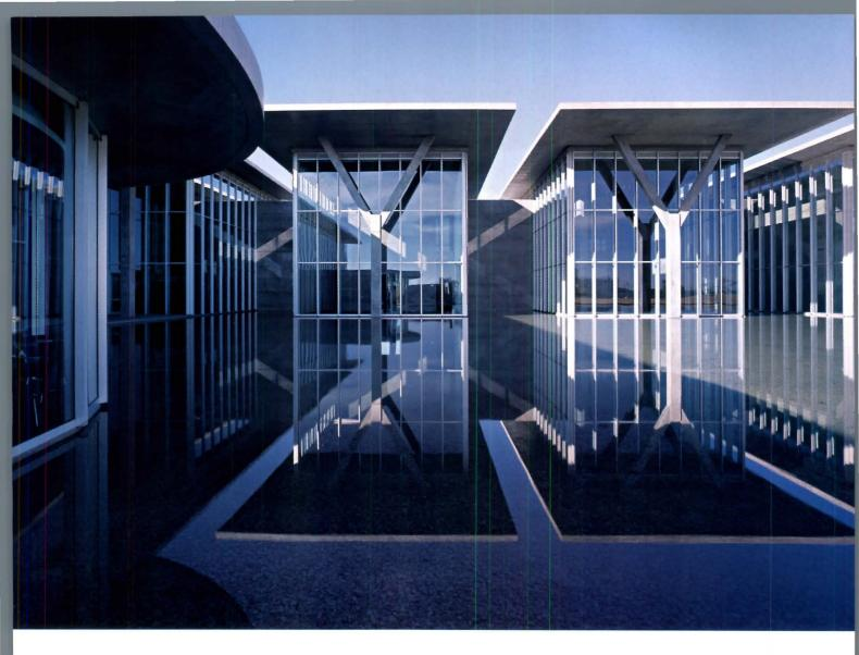
Ando designed the pavilions as long glass boxes with concrete cores (above). A long stair overlooking the pond helps animate the northernmost pavilion (right).
