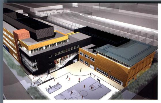
The tan-brick, whitetrimmed mass of the school takes up almost a whole city block (left). At the main entrance, the facade is composed of a handsome aluminum panel system and yellow curtain wall (below and opposite).
