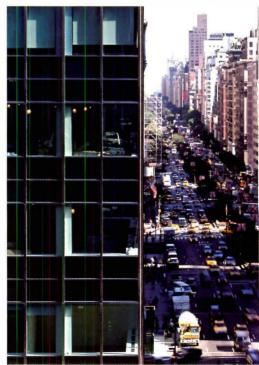
Whereas the wiredglass spandrel pan were originally divi into two parts with full mullion, now a nonfunctioning mul lion (above and left is applied to the pa els. The environme codes for energy us were waived so tha the same singlepaned glass could installed.
