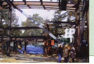
Eric Ko, principal with the project's structural engineer, Arup in San Francisco, noted that time savings are also realized, because unbonded braces can be bolted instead of welded. "Being able to bolt the connections cut 10 weeks off the steel-erection schedule and minimized the need for critical on-site welding," Ko says. Ko also noted that the unbonded braces can be made with circular tube steel that can present an attractive appearance if exposed.
