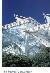
Center designed by Wimberly, Allison Tong and Goo. Features the largest suspended glass wall in the U.S. fabricated by Oldcastle Glass® in Stackwall."
