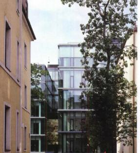
The architects and landscape designers wove a new courtyard into the office block (near left), creating a rich connection between old and new construction (far left). A double glass skin provides tempered air space between indoors and out (opposite, top).
