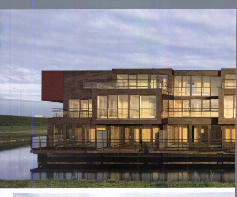
Attached houses face a lake (above), and single-family houses line a canal (below). Predesigned extensions (red-painted wood) cantilever on the second and third levels to take best advantage of views. Framed in metal, they easily attach to the concrete cores, which are covered in black slate shingles.
