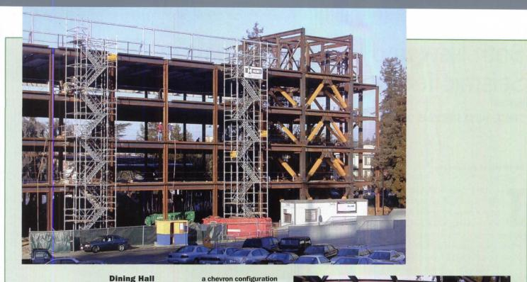
University of California, Berkeley Two kinds of unbonded braces were employed in this structure. The four-story office portion of the building has 16foot unbonded braces in a chevron configuration (above). In the 40-foottall dining hall (right), exposed unbonded braces as long as 37 feet were used. A typical brace would have been too large and ungainly to serve as a design element.
