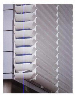
situations. They are manufactured from extruded aluminum sections and may be mounted at a fixed angle or with an adjustable manual or motorized system. Complete assemblies that incorporate walkways and supports together with handrail and other systems may be created using aluminum and steel components. Perforated fins and timber and glass options are also available. 44 20 8863 9111. Levolux, Middlesex, U.K. CIRCLE 235
