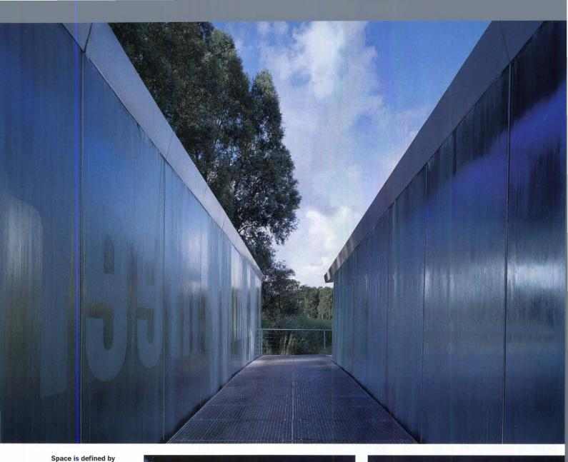
Space is derined by glass and water at the entry path (above) but flows freely around the exhibition pavilion (opposite, top). The glass sections of the entry canopy (near right and opposite, bottom) and main roof (far right) employ cables and suction cups engineered by the firm Octatube.
