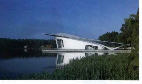
pair of supports. Where the two roofs meet, the architects inserted a walkway defined on either side by a glass wall animated by a sheet of sliding water, thereby creating a "water tunnel."
