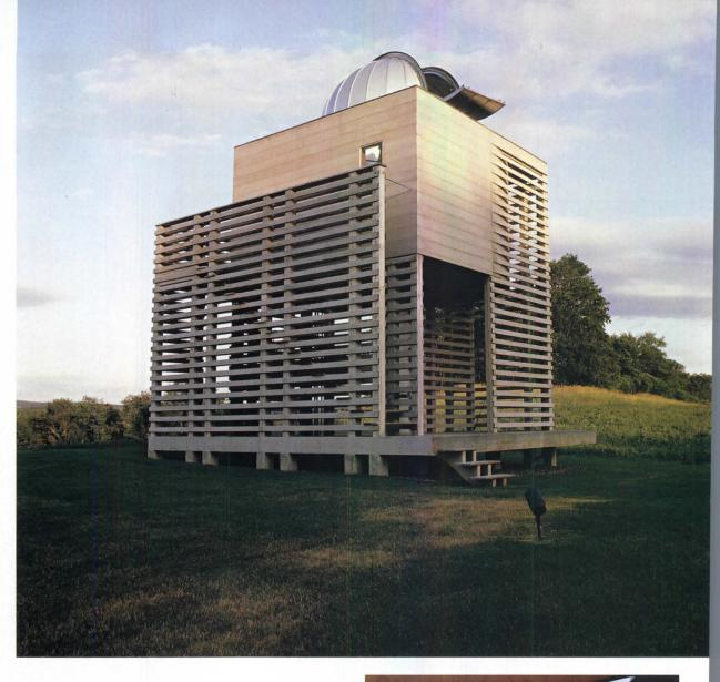
The viewing room (bottom) is sheathed in cedar siding and the tiny staircase and platform are wrapped with cedar posts and slats (right) spaced to echo the stair's riser dimensions.
