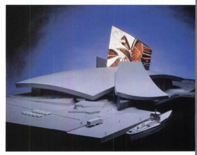
Libeskind first proposed thin-shell concrete roofs over a pancaked zigzag volume containing the exhibitions (opposite, bottom right). The shard idea was pared back (opposite, bottom left and middle, and viewed canal-side, this page), and the office later eliminated the thin curves of concrete and scrapped an ambitious program of artistdesigned gardens.
