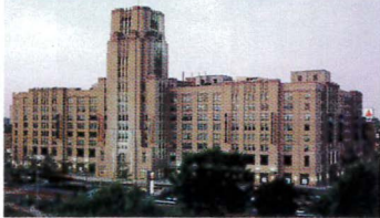
15,000 square feet of glass make up each atria of the Landmark Center.
