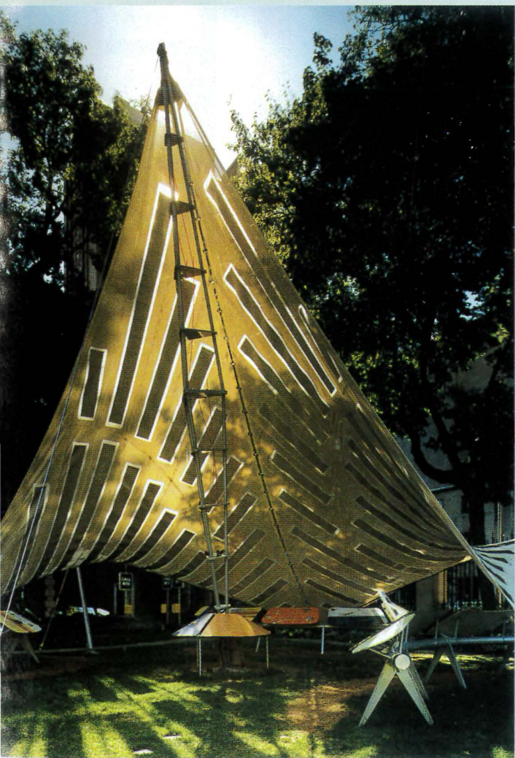
The tensile pavilion (above) at the Cooper-Hewitt exhibition had PVs laminated to the polyester fabric. The U.S. Army is investigating a field tent (right), called the TEMPER, an acronym for Tent Modular Personnel, which has PVs bonded to the fabric surface with pressure-sensitive adhesives.
