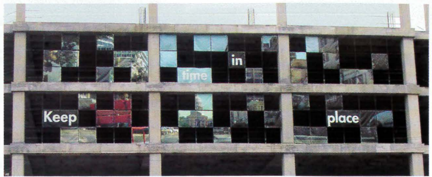
The fabric panels, with images and text printed on them through a digital process, are affixed to a cable system (below) on the concrete Intel structure in downtown Austin.
