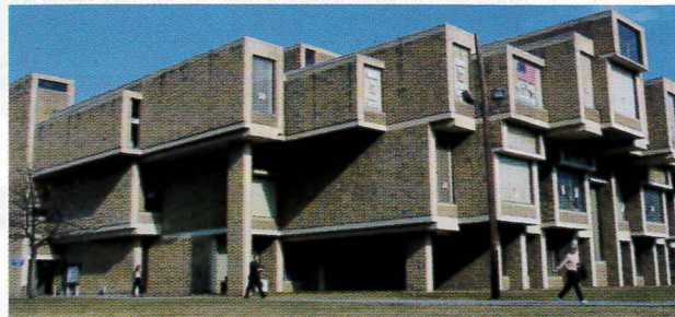
The Orange County Government Center by Paul Rudolph.
