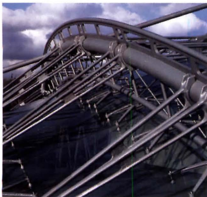
Tubular ribs frame the ticketing-level bubble (above) from the exterior (right), supporting armatures that attach glass by bolt-through connections.
