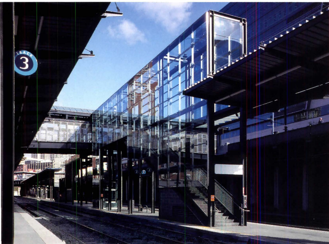
Light-filled glazed stairways and new platform roofs, designed by Otak, greet commuters on the Puget Sound region's new commuter-rail system at Seattle's King Street Station, which is shared with Amtrak.
