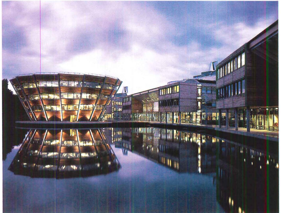
Tower-top cowlings, which can be seen above the buildings, help draw fresh air through the offices at the Jubilee Campus at Nottingham University in the U.K.
