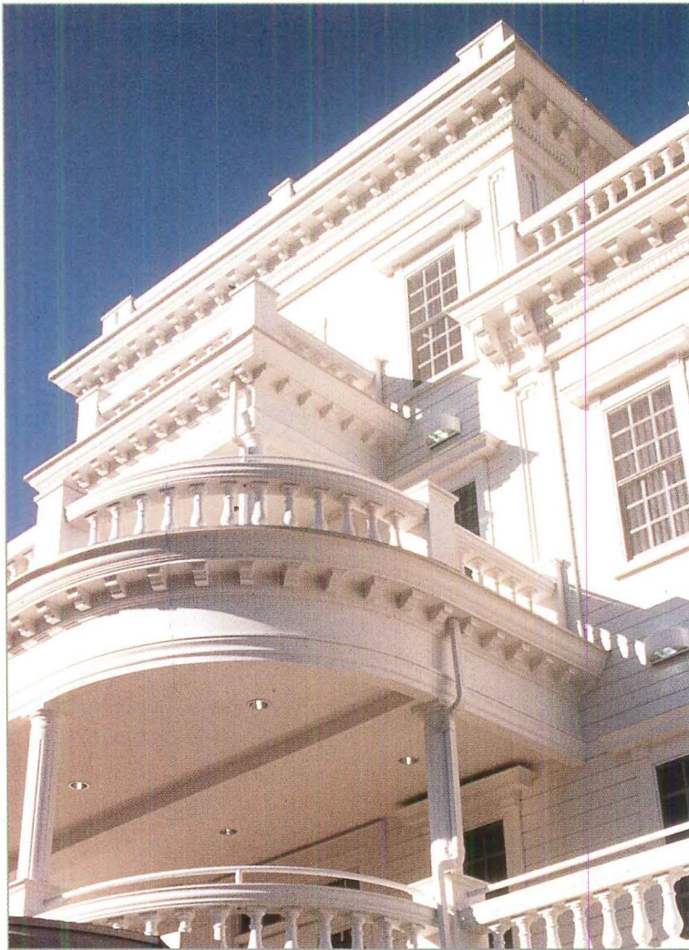
Incorporating dozens of urethane balustrade systems, corbels and brackets from Style Solutions, the Riverview Health Care Center resembles a stately hotel.
