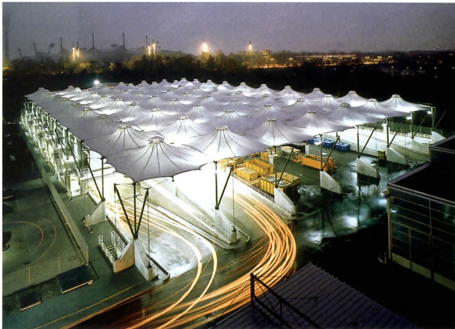
The AFA Carport in Munich illustrates one of the main advantages of fabric—large areas can be covered using a minimal amount of structural material.
