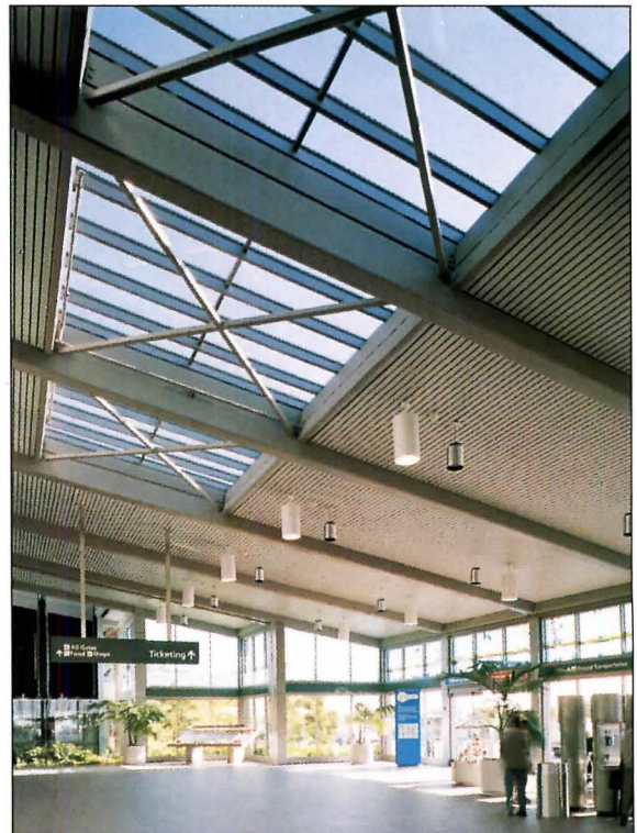
Photo: Sacramento International Airport, Terminal A Architect: Dreyfuss & Blackford Architects Photo: Cathy Kelly Architectural Photography A/D FIREFILM® II on structural steel.
