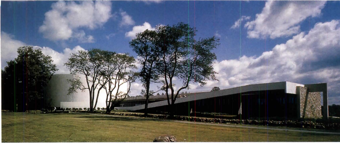
The endangered Cyclorama Building by Richard Neutra serves as the visitors' center at Gettysburg National Military Park.
