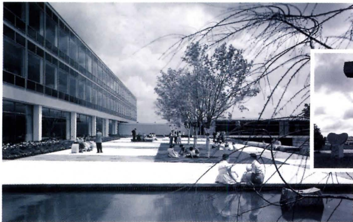
Wilde Building and courtyard slated for demolition, and sculpture to be sold.
