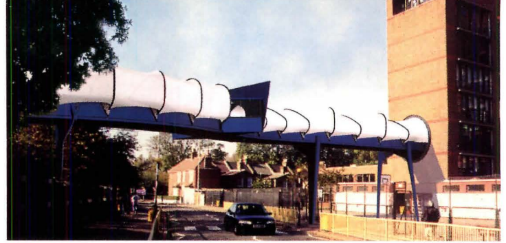
Fabric covers this footbridge by Birds Portchmouth Russum Architects.
