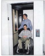
The Horizon is one of Concord's fully enclosed elevators. Its innovative cable hydraulic drive system delivers reliable, quiet & smooth operation while serving two to six stops. The Horizon is the ideal commercial accessibility solution for the physically disabled. Standard features include emergency battery powered door operation & lowering, a slack cable safety device, & emergency cab lighting. For information, please call 800-661-5112 or visit us at www.concordelevator.com
