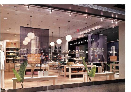
Display cubicles near the front entry "proscenium" (opposite and previous spread) are lighted with halogens. **Custom glass globe** pendants housing compact fluorescents (above and left) provide ambient light, while apothecary shelving units feature integrated T5 fluorescent lamps.
