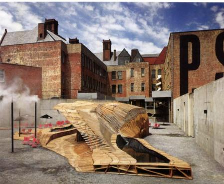
More than 6,000 cedar planks were used to build the dunescape in the courtyard of P.S. 1 (above). "CAT scan" drawings (right) were printed at jumbo size, laid out on the site, and used as templates for the actual structure.
