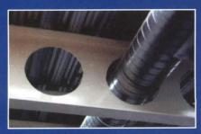
Electrical and mechanical services run through rather than under reducing floor to floor heights; therefore reducing costs of your structure.
