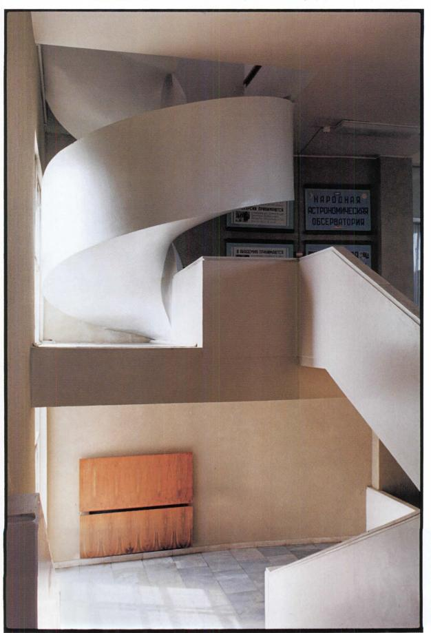
The spiral stairway leads to the observatory on the roof of the main block of the Cultural Center of the Proletariat district. Cast in one concrete pour, it has great sculptural presence and seems to float above the floor slab. It is one of the last buildings in Russia constructed in an uncompromisingly Modernist aesthetic.
