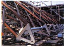
The MoMA arch began with four- to fiveinch diameter tubes (top). These were preassembled and lowered into place by crane. The arch rests on the ground and is tied to the museum wall (bottom).
