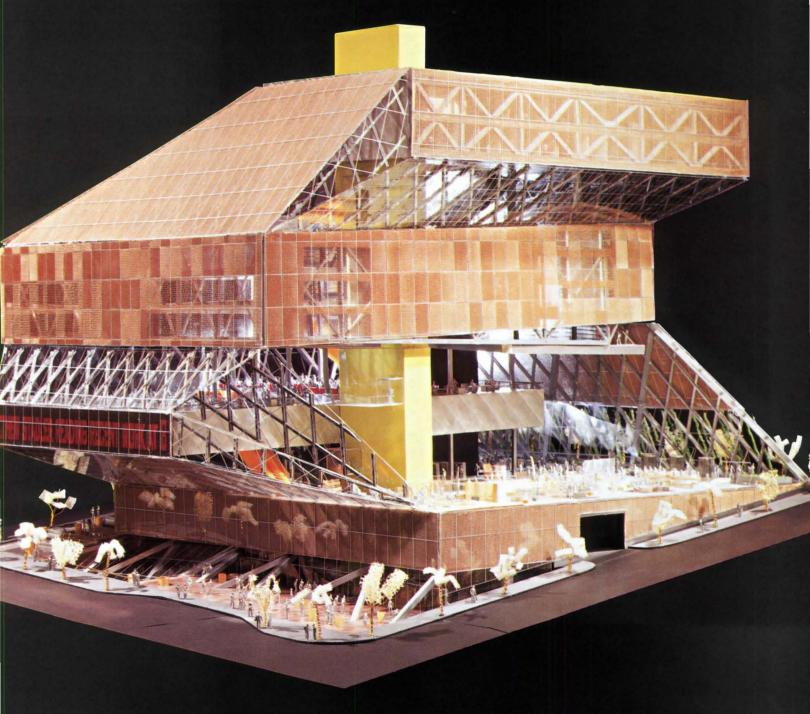
Blocks of floors shift toward views and light inside a diamond- patterned mesh woven by I-beams and steel tubes cloaked in a glass curtain wall. Alternating between five platforms (each devoted to a specific programmatic cluster) are four open spaces where patrons can meet, search the Web, or read.
