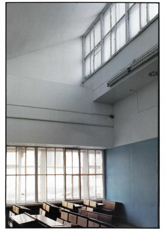
Now in an extreme state of disrepair, the dormitory building is undergoing a period of uncertainty. Three years ago the accommodation wing was completely gutted as if for renovation, but no work has been done, and with the windows missing the effects of the weather are hastening deterioration.
