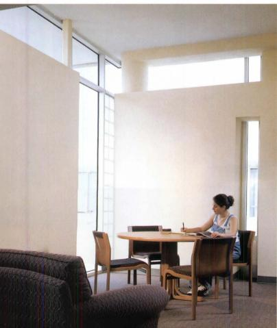
Window walls with clerestories and glass blocks flood bedrooms and study areas with daylight (left and below). These elements also vary the architectural geometry, an improvement on the "stacked box" housing the structure replaced.
