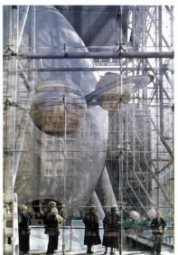
structural frame, were first modeled by Polshek in Microstation Modeler. a 3-D mechanical design software that complements Microstation, and transmitted via E-mail to TriPyramid of Westford, Mass., for fabrication. TriPyramid recreated the architects' Microstation models of cast spider fittings in SolidWorks, which drives the casting equipment. Similarly, TriPyramid redrew the machine-cut rod riggings from
