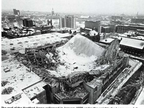
The roof of the Hartford Arena collapsed in January 1978 under the weight of a heavy snowfall.
