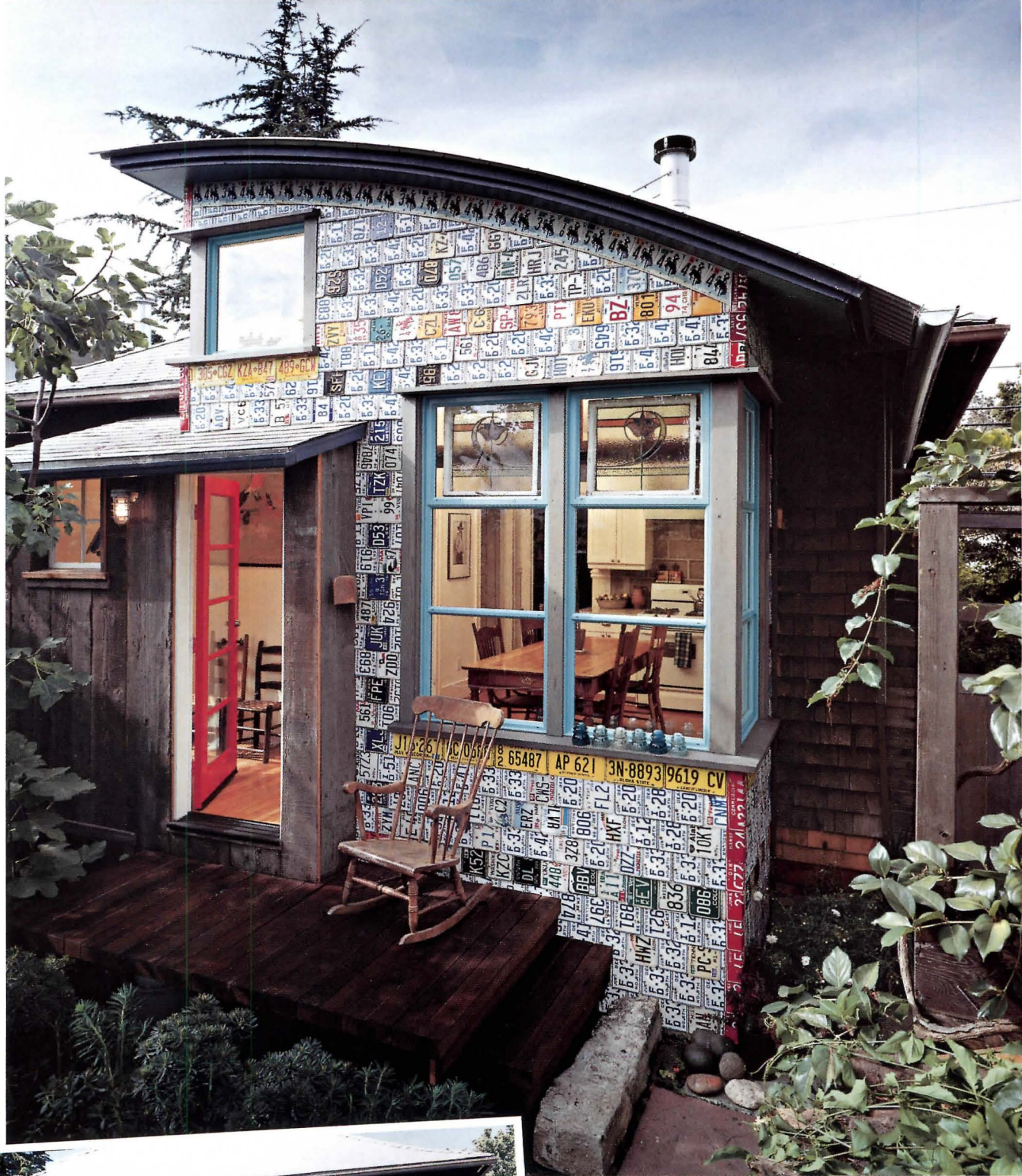
License-plate cladding on a new addition whimsically plays off the bungalow's original wood shakes, as seen before the renovation (below). The rear facade now opens the kitchen to light and views (right), raising the ceiling to create a clerestory beneath a new curving corrugated metal roof.
