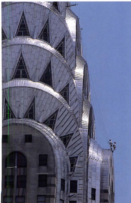
On the Chrysler Building, a Vertical Access rappeller uses high-tech investigation tools.
