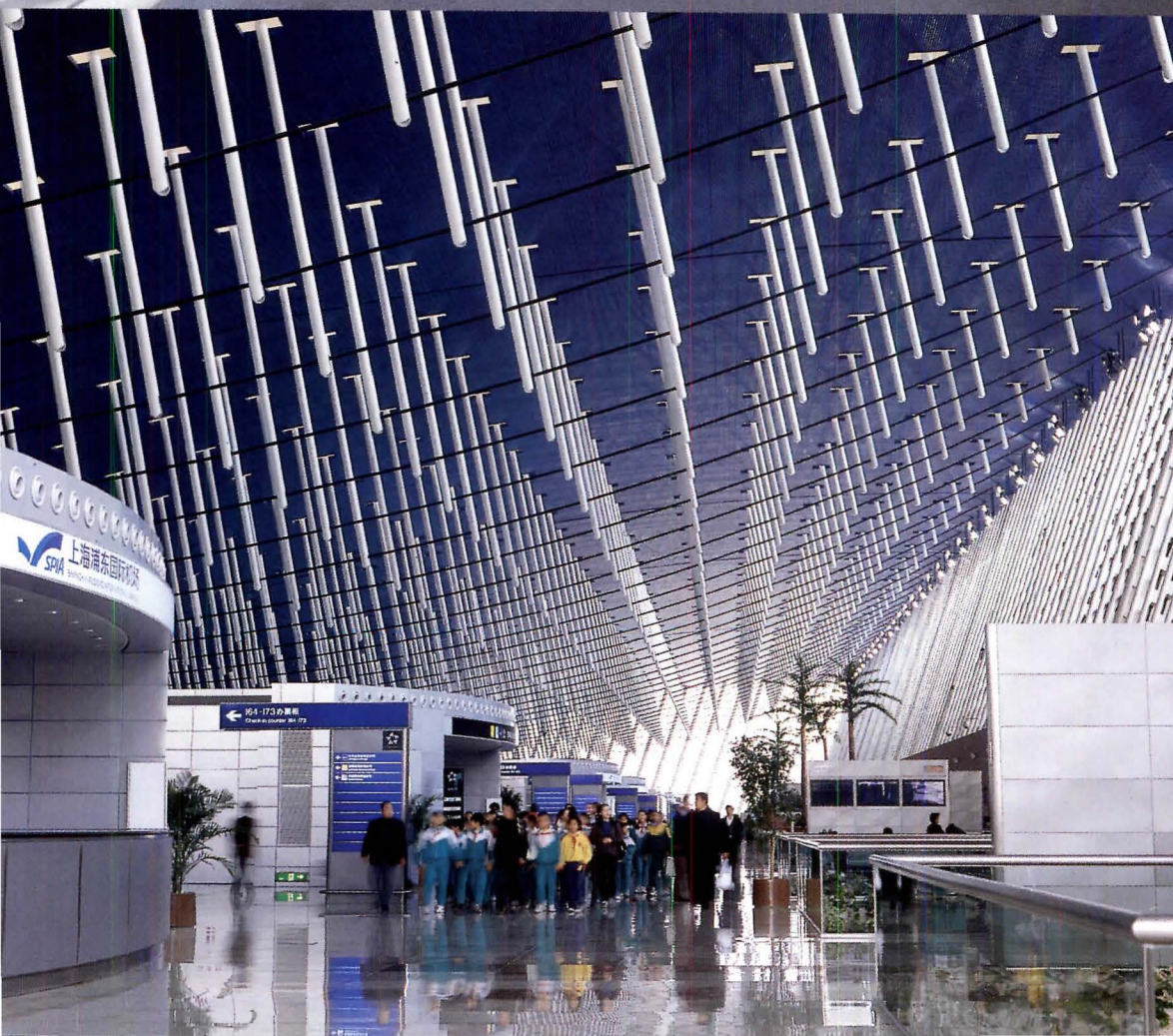
Throughout the project, roofs are prestressed parabolic trusses with lower chords that are cables.
