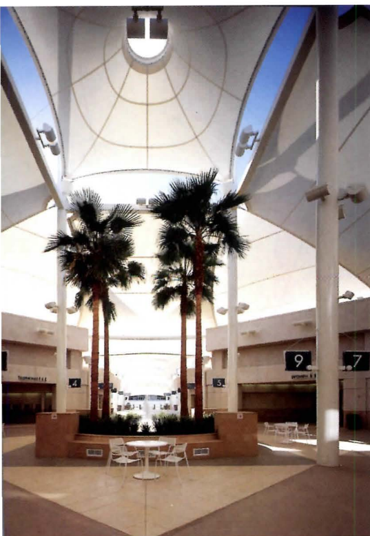
Teflon-coated fiberglass canopies help create shaded outdoor rooms at the new 11-gate concourse and terminal expansion at Palm Springs Airport, designed by Gensler.
