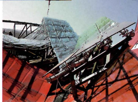
Clockwise: Detail of the metal connectors for the EMP; installation of the individual glass units. Below: Although CTEK's panels weigh 700-800 pounds each, they seem to float on air.
