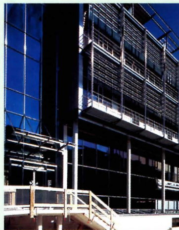
SBV Biel in Switzerland (above) uses prismatic elements placed high in the window bays. They are a striking visual addition to the building's facade and reduce glare and veiling reflections on the interior, while leaving views through the lower, clear glazing undisturbed. A detail (right) shows how the prisms are attached to the curtain wall.
