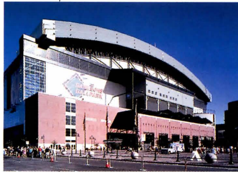
Phoenix's Bank One Ballpark by Ellerbe Becket was the first in the nation to use a retractable roof.
