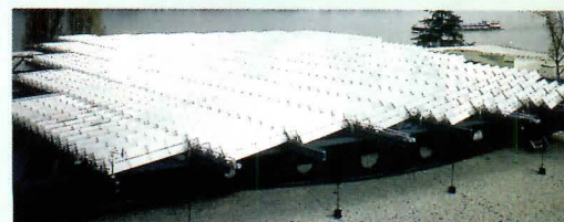
The roof of the German Parliament building in Bonn has adjustable prisms on top that redirect light into the main hall (below), allowing television broadcasts to be shot without the use of electric lights.
