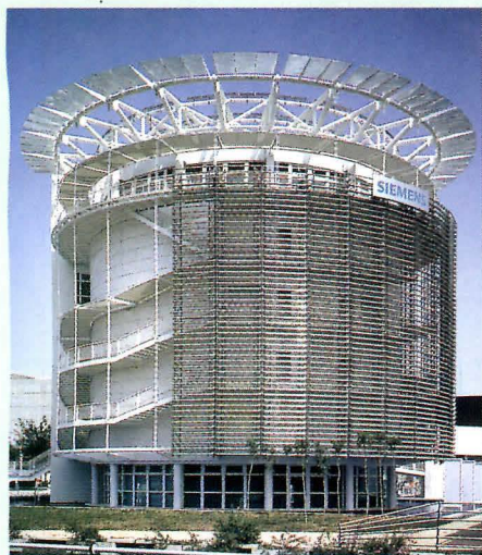
The Siemens Pavilion (above), built for Sevilla, Spain's 1992 exposition, uses a seasonally adjusted prismatic sunscreen to protect the building from the sun. The 3M Corporation's Austin Center uses a mirror system (right, top, and middle) and the company's prismatic film to light the building's atrium (bottom right).
