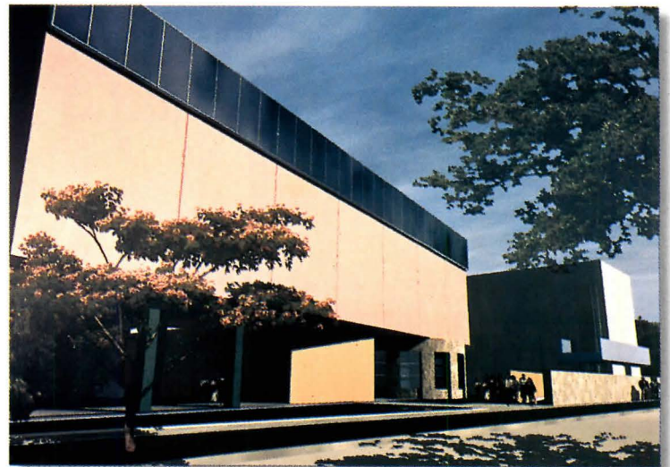
Isozaki's addition to the Bass Museum should be completed this year.
