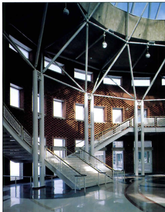
Photo: Chicago State University, Rotunda Hall Architect: Harry Weese Associates, Johnson & Lee Photo By: Ken Kavana A/D FIREFILM® on structural steel
