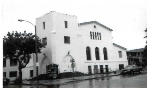
Stealth Network Technologies' fiberglass shielding system provided enclosure for wireless communication equipment atop a church in Monrovia, California (before, left, and after, above).
