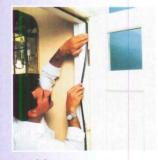
lem: The Infiltration of Sound, Smoke, Drafts, and Light. Solution: Pemko's State of the Art, Self-Adhesive Door Gasketing, SiliconSeal™ and PemkoPrene™ - Fire Labeled (UL10B, UBC7.2 Positive Pressure) and Smoke Labeled.
