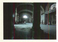
windowpanes have been broken, the iron roof has gotten rusty, and glass and plaster have piled up.
