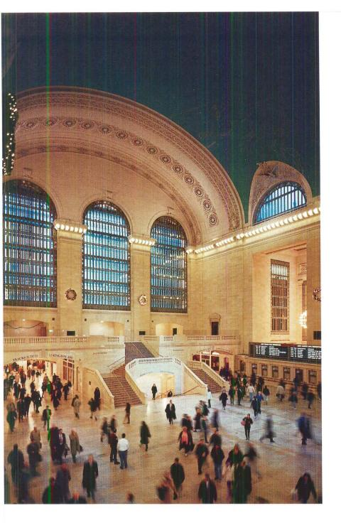
The terminal's arched windows (left and below) each measure 33 by 60 feet and form a double skin of glass. Glass walkways run between the two transparent skins, connecting offices on either side. A new east stair (left) stands where the Kodak sign used to be and provides access up to restaurants on the
