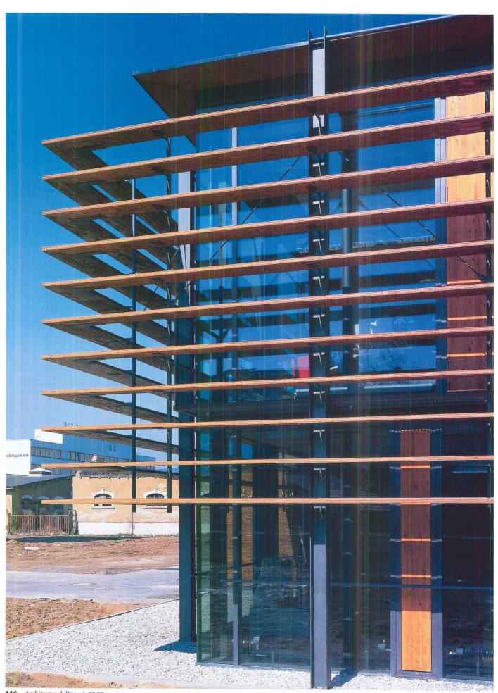
A steel structure supports the curtain wall, as well as Nordic-pine plywood louvers, which allow for transparency while shading the interior (right, below, and opposite). Louvers are set two feet from the face of the glass to provide minimum width for a second-story fire escape. Lamott gave the louvers openended fins (below and right), instead of wrapping the entire building. Befitting a library, the interior is legible from outside.
