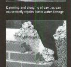
The Mortar Net Drainage System allows water to maintain a path of exit to the weeps, preventing damage caused by the blockage of weep holes.
