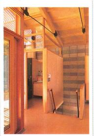
place materials in standard modules—maple plywood sheets and integrally colored concrete masonry blocks—to form open yet ordered, light-filled spaces. (With Zenlike precision, even the shower's black ceramic tiles were laid out so that no piece had to be cut.)
