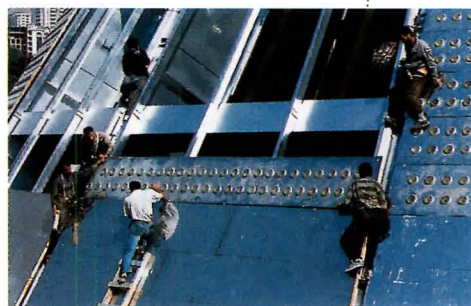
The main facade of the 250,000-square-foot International Conference Center in Teheran (above). Local laborers work on the dome, whose panels were fitted with 40,000 glass cylinders (left).
