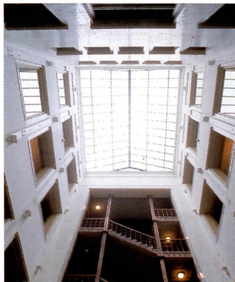
Restoring the original light courts in the 103-year-old Portland (Oregon) City Hall included exposing the roof glazing and the white glazed-brick walls. The courts bring daylight into the offices and create a central meeting place.
