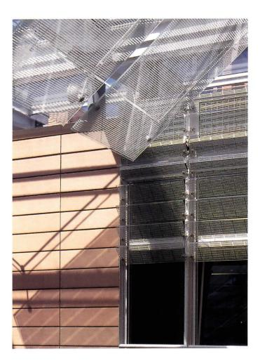
Plans (opposite) show how nearly every building element has been carved away to reveal itself on the exterior. Following German building regulations, the majority of work spaces include an operable window. Sunlight from the atrium's all-glass roof is diffused through milky glass panels fixed at an angle (left). Additional fins are mounted at the office windows that face the atrium. The solid cladding is terra cotta.
