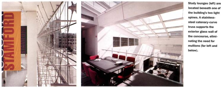
located beneath one of the building's two light spines. A stainlesssteel catenary-curve truss supports the exterior glass wall of the concourse, eliminating the need for mullions (far left and
