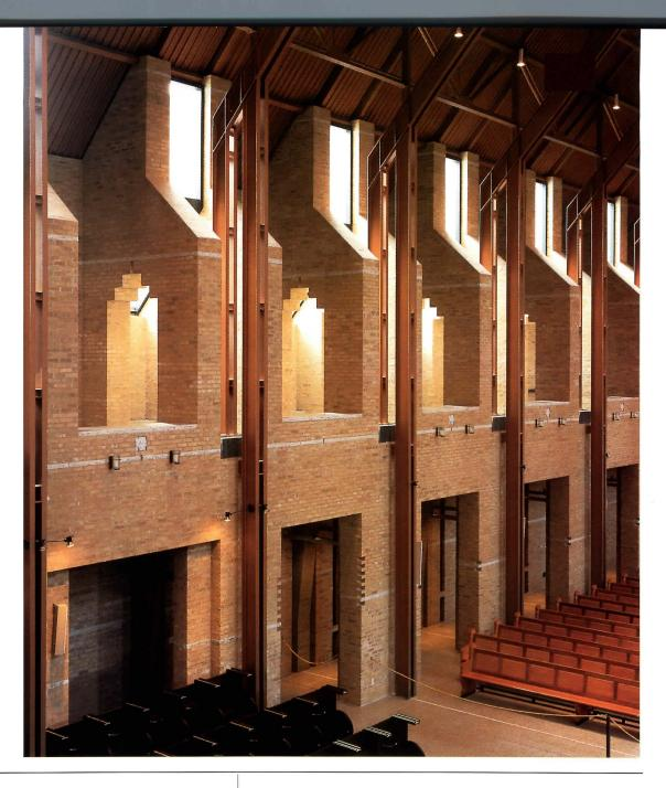
The church features an internal buttressing network fashioned from steel, supporting a simple peaked roof.
