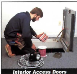
Interior Access Doors
