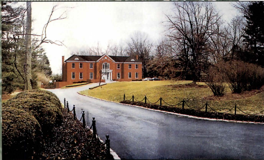
Private residence by Mackey Mitchell Associates, modeled in Alias Upfront and rendered in Photoshop by Paul Wuennenberg
