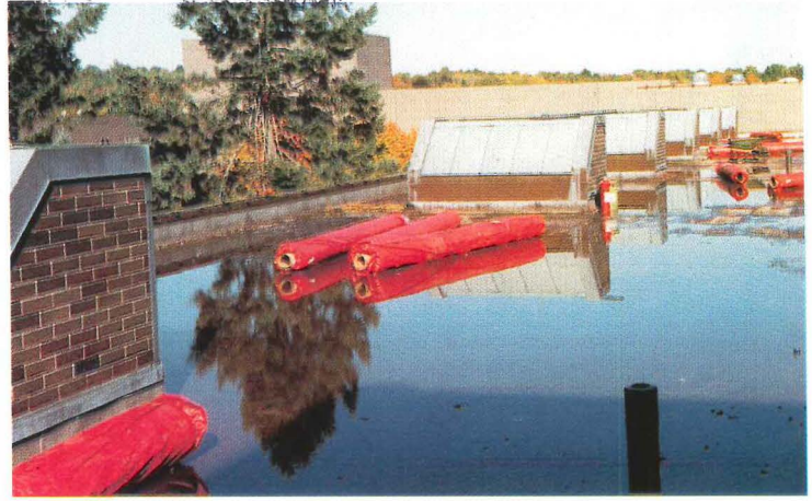
Pipe penetrations at curbs (left) are a reroofer's nightmare, only made worse by the wiring. An independent roof inspector can call attention to such contrary-to-specs conditions as new roof materials stored where they can get wet (right).
