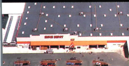
Hi-Tuff/EP works at Home Depot.
