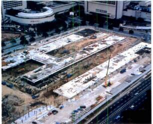
In the top-down construction used at the Singapore International Convention and Exhibition Center (left and drawing above), the ground-floor slab was built in an E shape, which allowed excavation to the first basement level to be done mostly in the open
