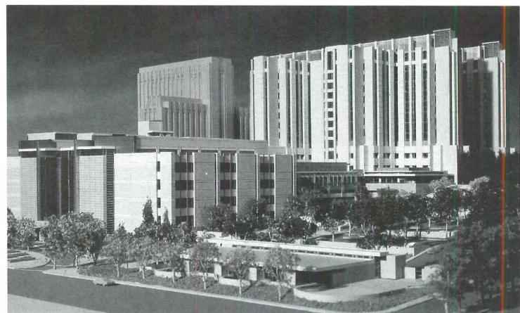
Lee, Burkhart, Liu's original design (above) for a new Los Angeles County-University of Southern California Medical
