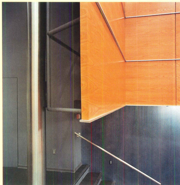
upper walls, refinished in aluminum-splined oak-faced panels, wrap the stage, forming a proscenium (4). Over the stage, expanded-metal fabric conceals speakers and theater lights (2).
