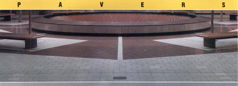
Five new porcelain pavers with water absorption rates of almost 0%. And breaking strengths that double the ANSI standards.
