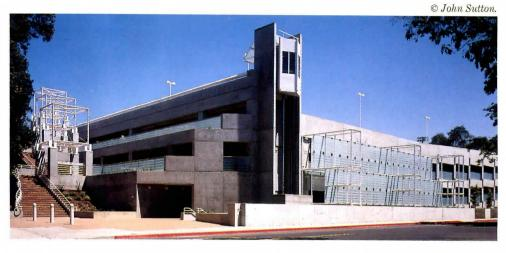
Cast-in-place construction met strict needs at the University of California, Davis, Quad District Parking Structure (HGHB Architects and Forell/Elsesser, engineer). 36-in. deep post-tensioned beams span 60 ft, keeping floor-to-floor at 10 ft. Inverted Tshaped shear walls and concrete ductile moment frames resist seismic forces.
