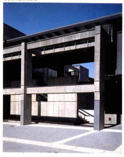
Kieran Timberlake & Harris used smooth forms for concrete at the University Center at East Stroudsburg University (RECORD, October 1993, pages 110-111). Granite coping stones protect horizontal surfaces exposed to weather.
