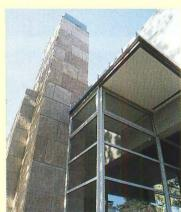
Similar details ease transitions between standard steel window walls and wood (top), metal (middle), and stone (bottom).
