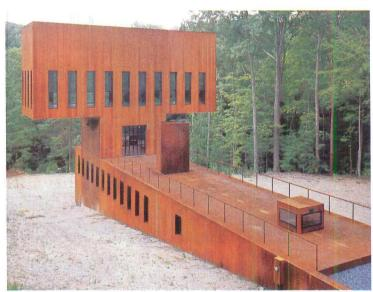
The 1/4-inch-thick steel exterior shell was prefabricated in six parts and then transported to the site, where it was assembled on top of concrete foundations (photo below left). The steel's nickel and chromium finish has oxidized to a vibrant rust color.
