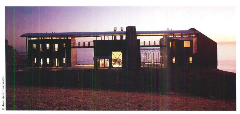
Heavy winds, the weight of up to 300 guests, and brush fires were among the design problems. An extra-heavy structure and a galvanized-steel roof over rigid insulation were the solutions.
