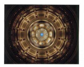
The lower rotunda (upper left) is illuminated by uplighting through the glass floor, new PAR30 uplights recessed into the floor, existing architectural brackets, and spill from the flag cases and portrait lighting. The upper rotunda (above) is washed by concealed PAR30s and metal-halide spots. The restored architectural wall brackets and floor uplighting wash the walls on the second floor of the rotunda. Existing harps (lower left) light a stairway.
