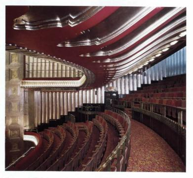
Dramatic lighting makes full play of the Savoy's aluminumleaf decoration. Long-life tungsten lamps are used in the ornate ceiling coffers over the stage and along the balcony fronts, while cold cathode gently highlights the edges of the balcony ceilings. All the house lighting is controlled by a single dimming system.
