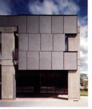
To economically add lounges, offices, and food-service areas to an existing student center, Kieran, Timberlake & Harris wrapped the brick-clad original with a small addition to the south and a larger addition to the north (drawings above). The wall expresses its layering of cast-in-place concrete frame (which forms an arcade on the north side, opposite and left), suspended open-joint granite panels, and windows set in the backup wall (above).
