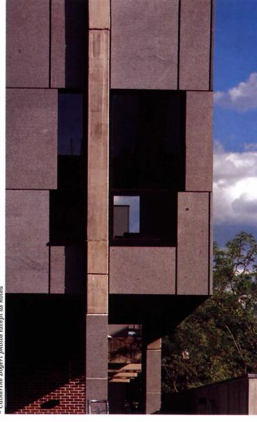
2-in. clear space between the suspended panels and the backup. It's not quite a cavity wall, as commonly seen in brick and block construction, nor is it quite the pressure-equalized rainscreen wall seen on highly engineered curtain-wall systems. This idea is called a "ventilated wall" in Europe, where it is more widely used, though systems are now available here (you can buy clip systems for stone or tile panels). "It's a step toward the sealant-free building," says Stephen Kieran.
