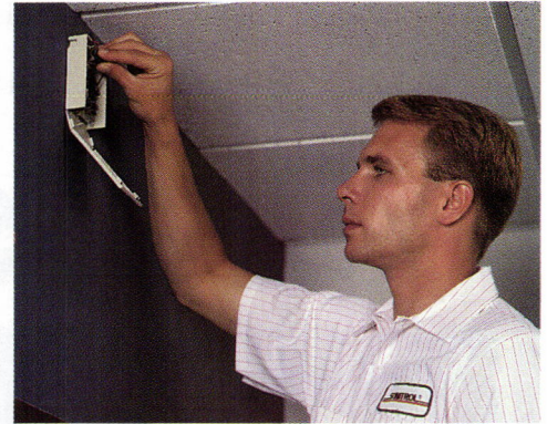
Below: A wall-mounted audio sensor detects the presence of unauthorized persons in a school and reports to a security monitor point. Card-access systems (not shown), frequently used for school labs, record time of entry and owner of the card.
