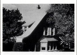
**344.** Reroof option. The Homecrest aluminum shingle, a new style, has an authentic slate, shingle, or tile texture, offered in five colors. The lightweight, individually fastened pieces are installed from the ridge down. Alcoa Building Products, Sidney, Ohio. ■
