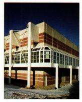
Reynobond®FR Aluminum Composite Panels were utilized as spandrel panels, fascia, soffit, column covers & truss beam wrap on the M.I.T. Lincoln Laboratory Facility. Reynobond®FR is the only solid thermoplastic core composite panel whose core material is categorically inert, non-toxic & fire resistant. Case history available with supporting data. Reynolds Metals Co., P.O. Box 27003, Richmond, VA 23261. 804-281-3629.
