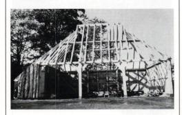
**343. Traditional English.** Eighteen different one- and two-story structures—based on historic British construction—are offered in pre-cut kit form. The post-and-beam frame is made of green well-boxed oak heartwood, with mortise-and-tenon joints secured with pegs. Options include crown-post roof, jowl posts, and mullioned windows. Open bays permit flexible partitioning. English Heritage Oak Buildings, Wadhurst, England.
