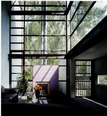
Norten ganged an interior and exterior staircase along the front of the Ortiz house, buffering living spaces from the busy street. Slot windows on the ground floor block views of passing cars but frame trees in the distance. Varnished steel I-beams bracket the two-story living room and help support the curved poured-concrete ceiling (bottom left and opposite).
