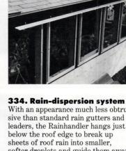
With an appearance much less obtrusive than standard rain gutters and leaders, the Rainhandler hangs just below the roof edge to break up sheets of roof rain into smaller, softer droplets and guide them away from the foundation. The louvered disperser is made of aluminum, and is said not to clog with leaves or form ice dams. A demonstration video-tape is available free to architects. Savetime Corp., Bridgeport, Conn.
