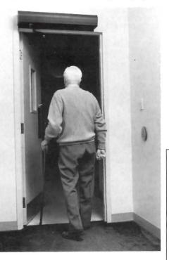
16. Door operator. Gemini GT operators rovide the option of both manual and autoatic access. They are suggested as an conomical retrofit (under \$1,000) to make for accessible to the elderly and handiapped. All components are surface mounted or easy installation on existing doors. Both old-open delay and opening speed are adstable. Gyro Tech, Inc.
